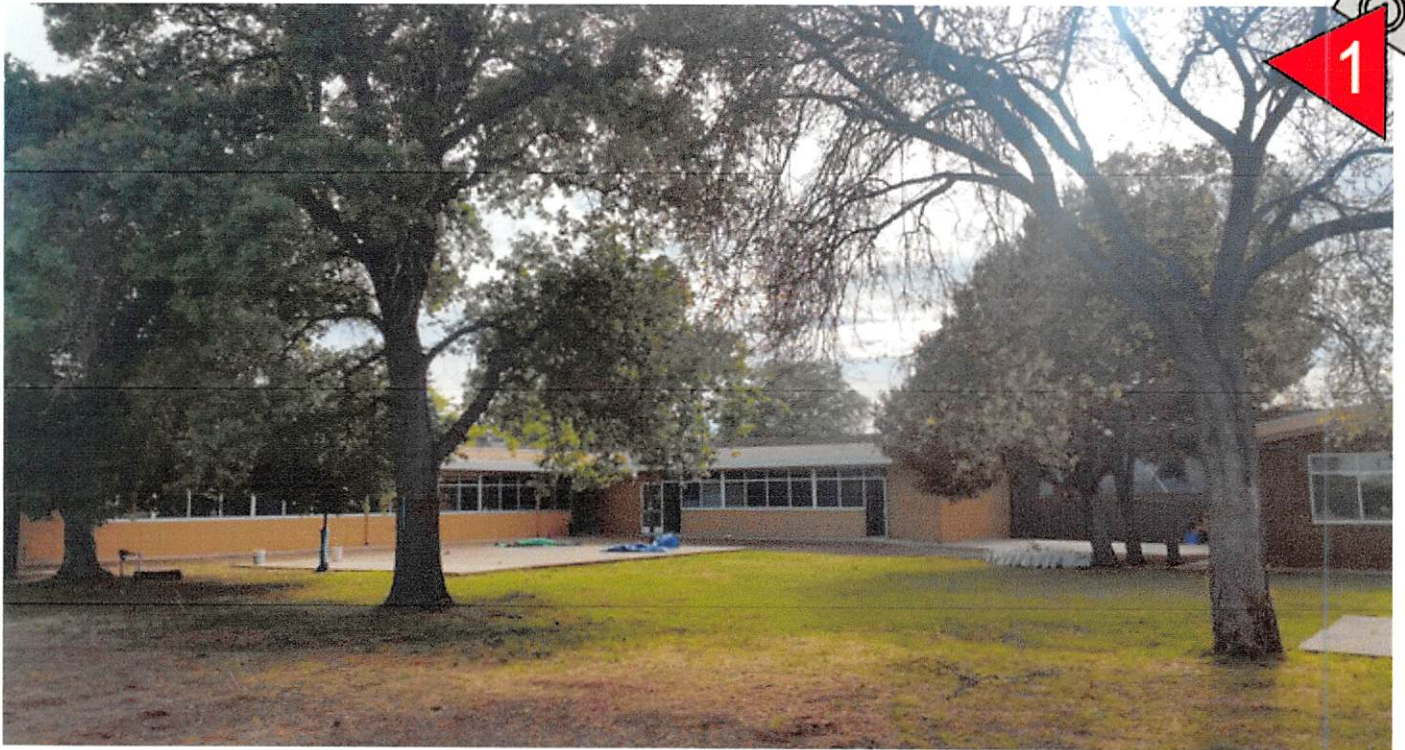
From northeast corner looking into project site
