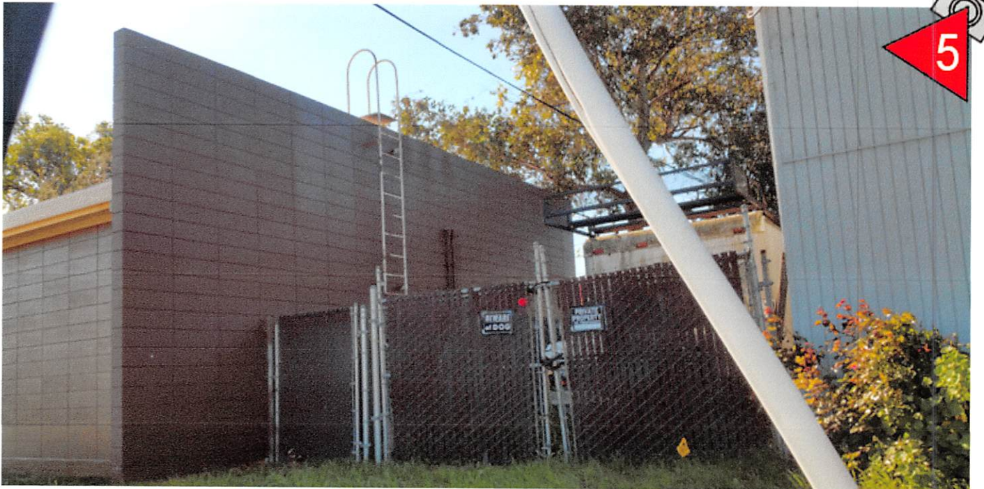
Close-up of northwest side of project site
