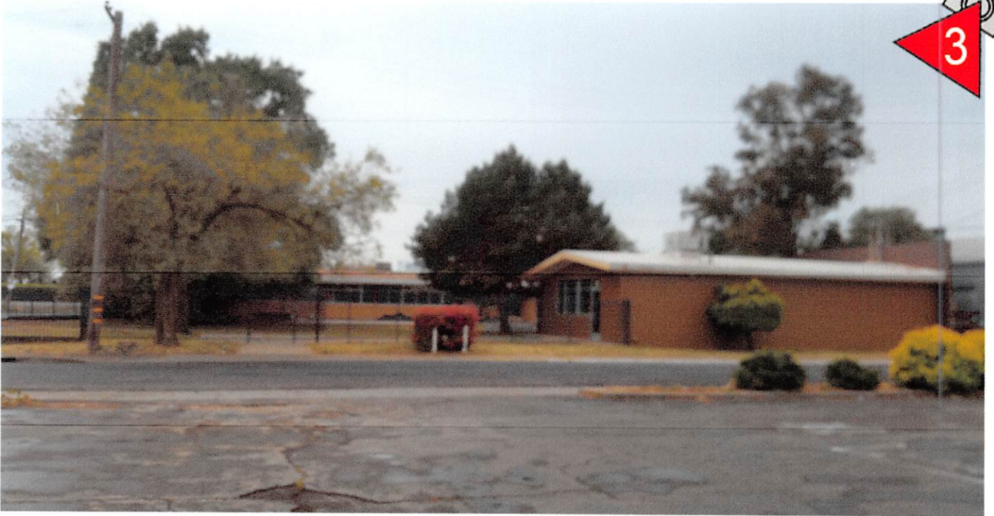
North side of project site
